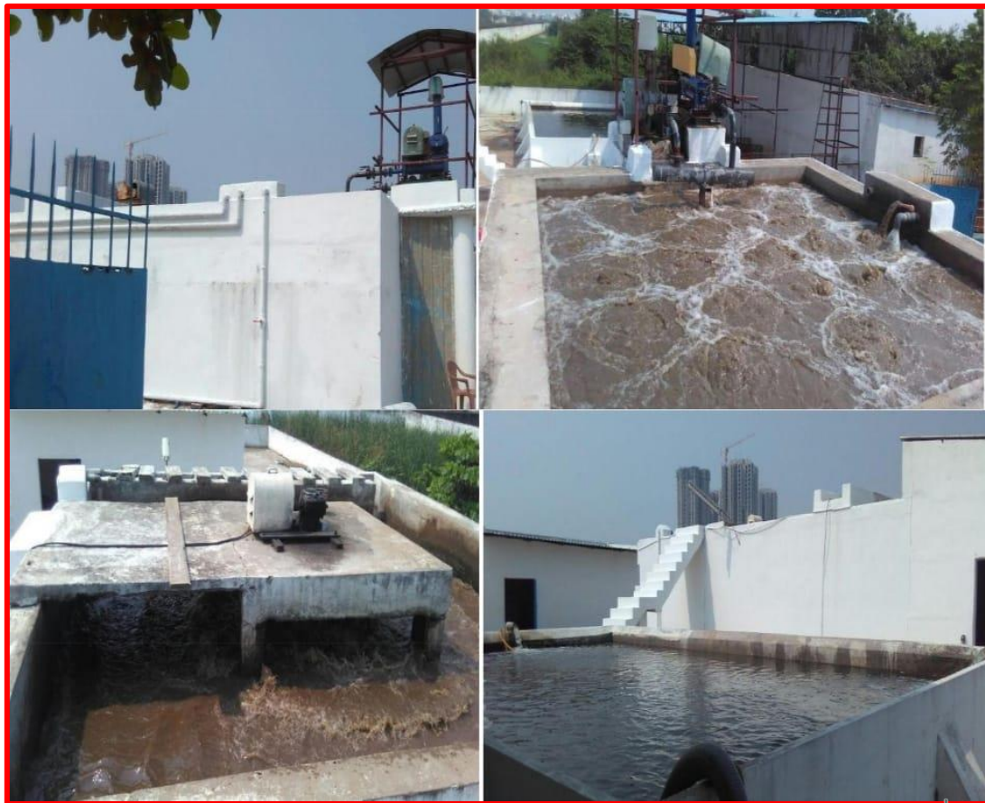
SEWAGE TREATMENT PLANT
